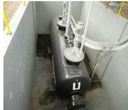
Fotografía 12: Closed Drain
