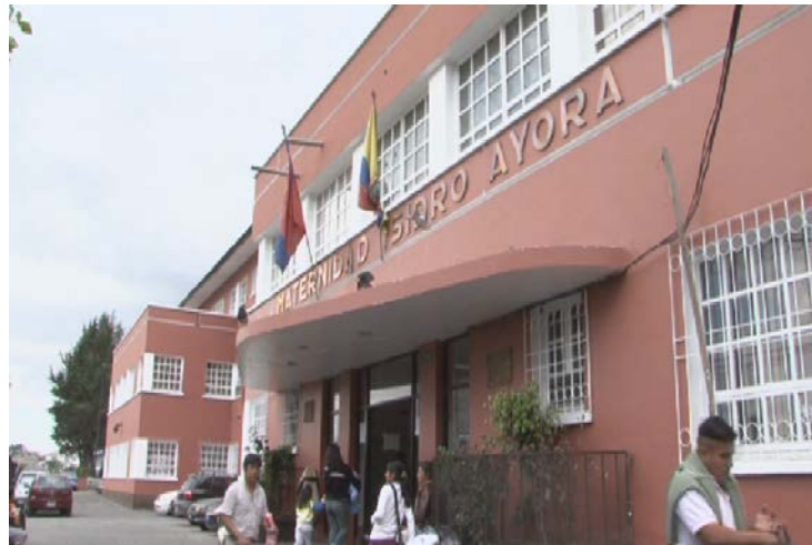
HOSPITAL GINECO-OBSTÉTRICO "ISIDRO AYORA".
